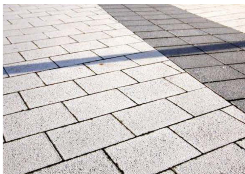
Concrete block pavers with paving bands
