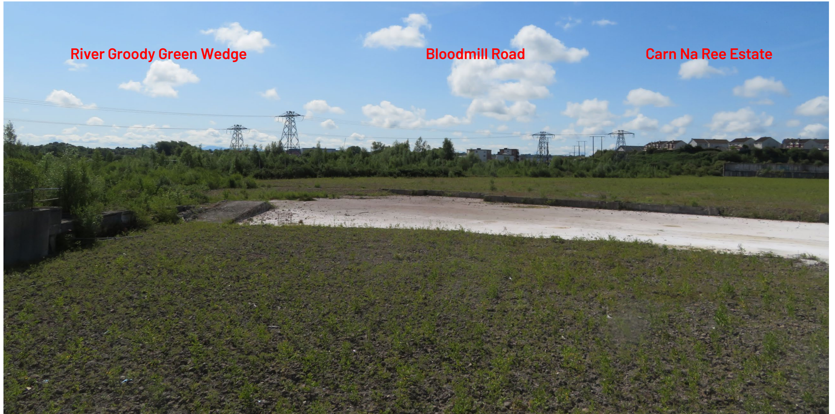
Figure 10 : View from within site facing south with Chesterfield and Carn Na Ree residential estates in the background.
