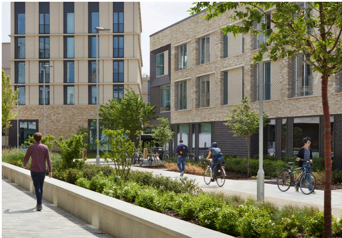
Figure 24 : Raised plating provides a buffer to ground floor residences
