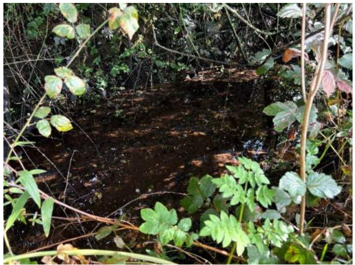
Figure 2-2: Existing Open Drain
